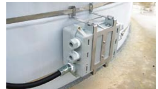
Sensor unit installation
